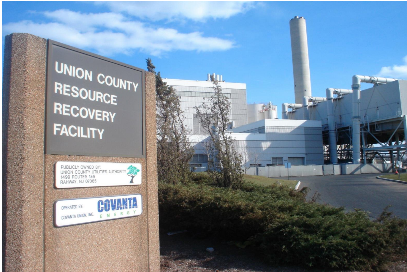
UNION COUNTY RESOURCE RECOVERY FACILITY
